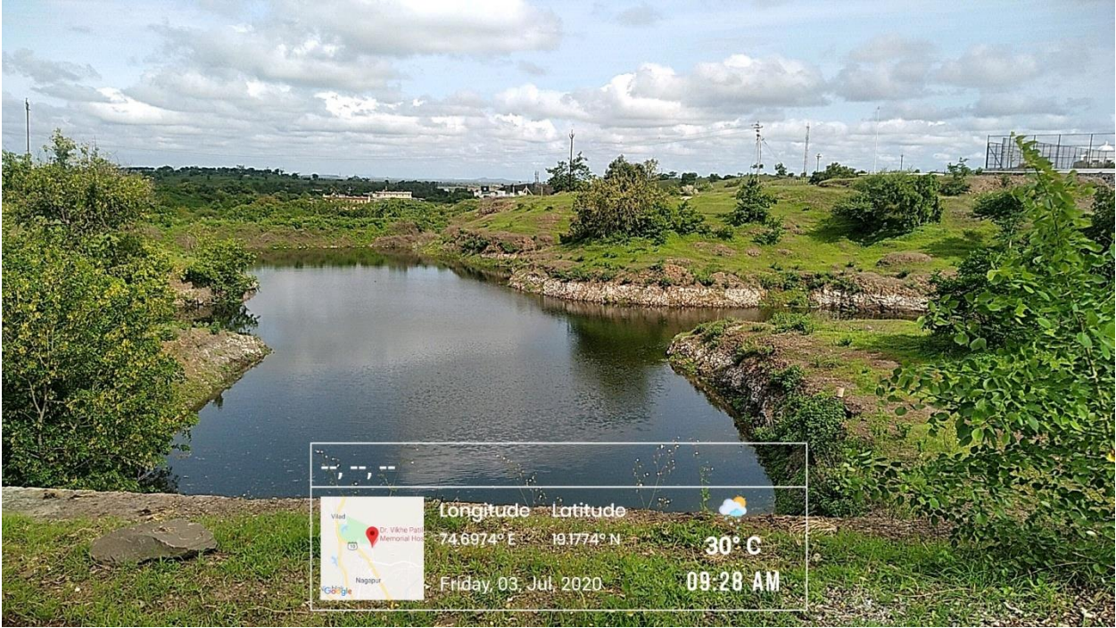
Check Dam No.2
